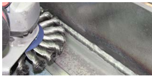
Weld seam cleaning with a round knotted brush
