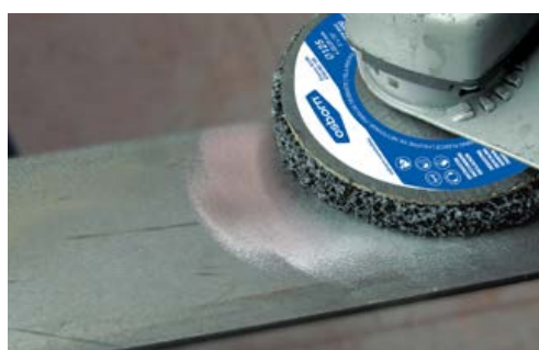
Cleaning/descaling steel surface with the coarse cleaning fleece.
